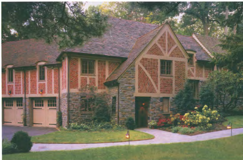
Peter Zimmerman Architects added 3,000 sq.ft. to a ca. 1935 Tudor-influenced residence in Bryn Mawr, PA, in order to accommodate a growing family. The addition comprised a family entry, three-car garage, family dining room and three new bedrooms and baths.
