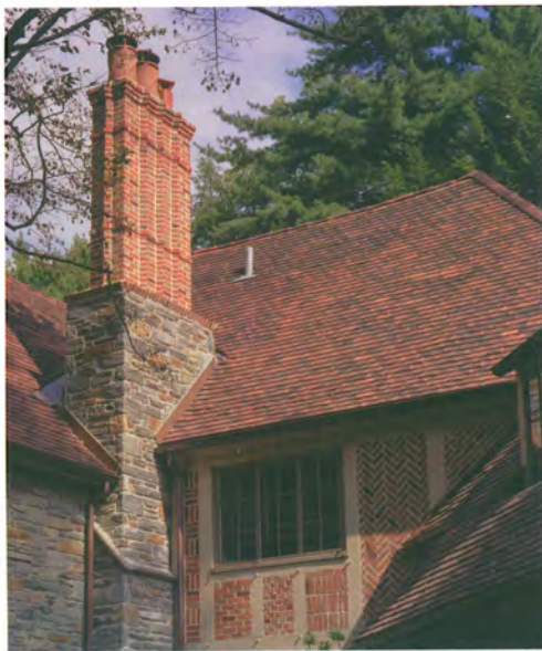
The brick patterning of the chimney was designed to complement the existing chimneys. (Glen-Gery and Boral Bricks, Inc., provided the brick.) The composition of rooflines was configured to provide a constantly changing play of light and shade on the exterior materials of the house. The custom Ludowici roof tile has yet to gain the mossy patina found on the existing roof.
